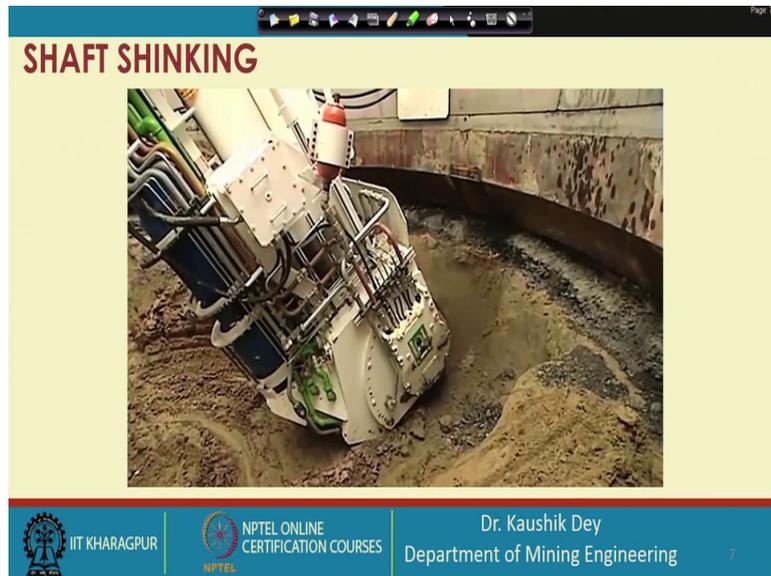
So, after creating and opening up a significant distance a significant depth the lowering of the side wall supports has to be carried out.
