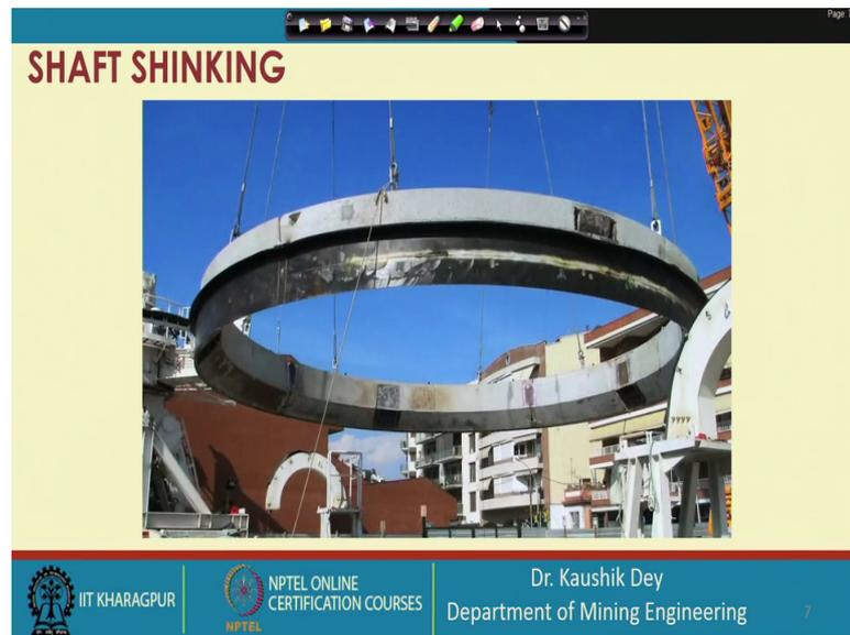
Strand wires are connected to pockets in the cutting edge. The numbers of strands corresponds to the total weight of the shaft.
