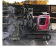
Hydro removal equipment
