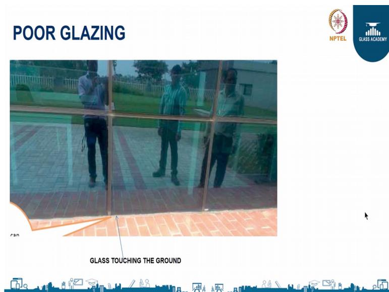
You can see glass is touching the ground on that surface and there is no space for expansion and contraction. Glass in this photograph you can see glass is directly grouted on the ground without any gasket.
