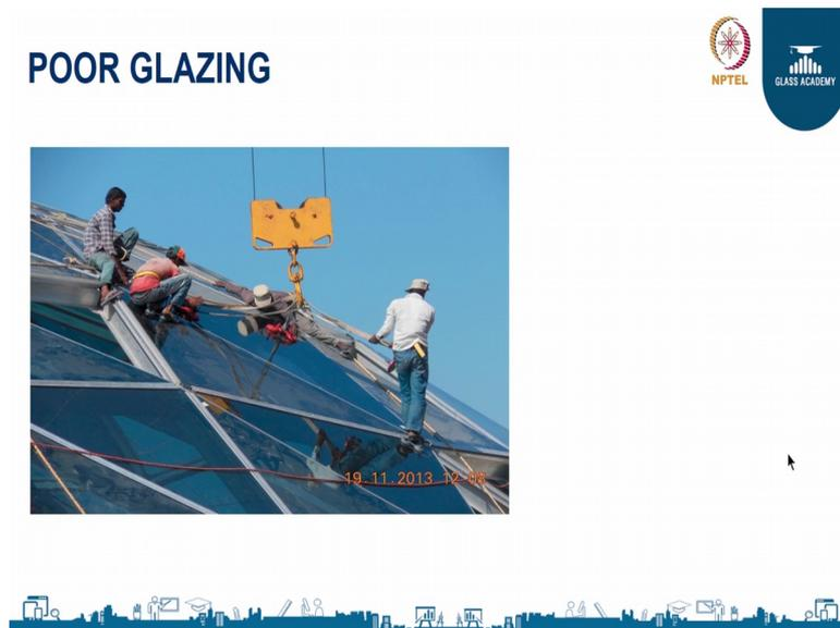
Poor glazing you can see the glass people are moving on the edge of the glass surface, which will also lead to breakage of the glass surface in future.
