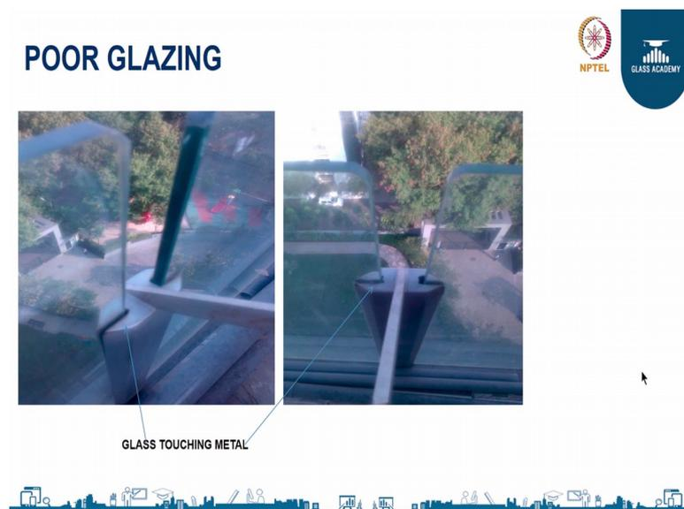
And this you can see the glass is touching the metal in that photographs. So, there is no space for expansion and contraction of that glasses which will lead to breakage.
