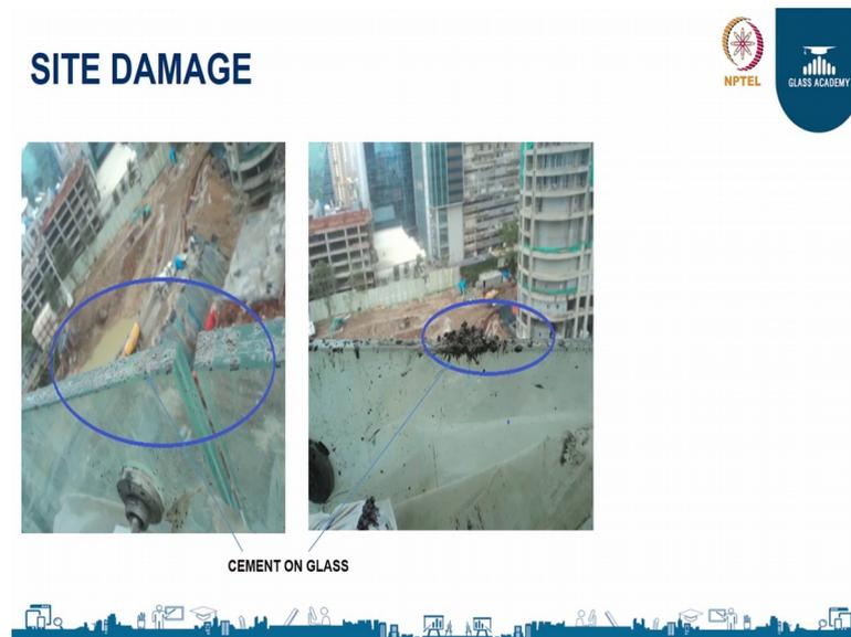
You can see some photographs of the site where the cement is there on the edge of the glasses. So, in order to remove the cements normally what happens is people will use metals or some abrasive material to remove this cement from the surface which will damage the glass surface and it might create crack in future.
