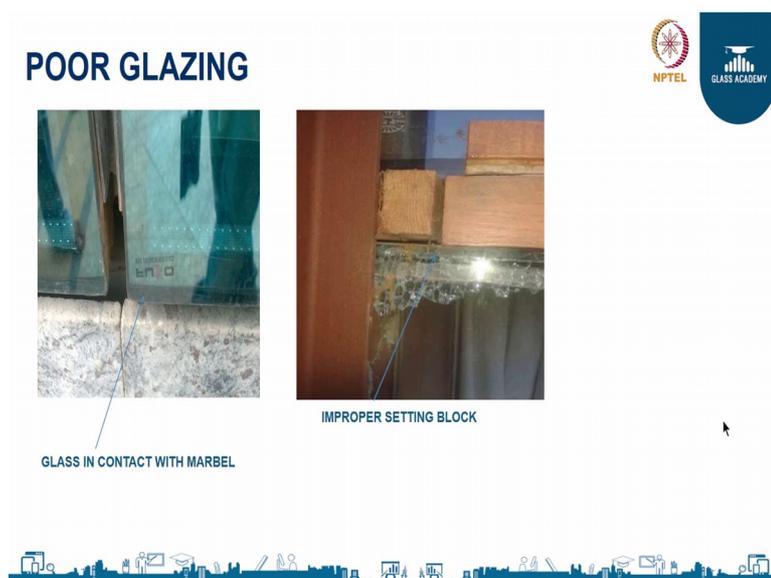
You can see in the left hand side glass in contact with the marble so, it will break eventually. See in the in the right hand side in monitor, you can see the setting block has come down and creating a pointed load at that point and the glass is broken.
