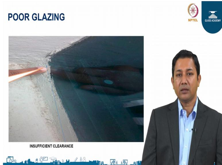
You can see the glass is supported with the plasters there is no clearance for the glass for expansion and contraction, so which will lead to breakage.
