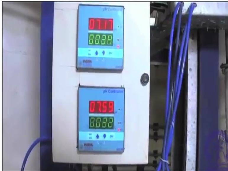
Groundnut De oiled cake is a byproduct of the agro processing industry; this product is rich in nitrogen, minerals and vitamins. Our lab scale experiments have shown that addition of groundnut De oiled cake to the media have significantly improved the hydrogen production. Upon thorough mixing it was essential to adjust the pH of the media, the plant is equipped with a pH dosing and a control system the final pH of the media was adjusted to 7.
