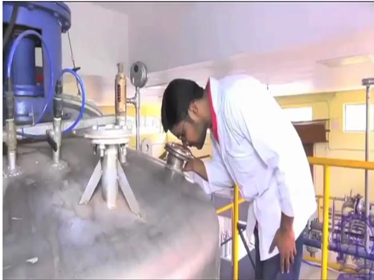
Constant sampling of the 10 meter cube reactor is done to monitor parameters such as pH, COD and the volatile fatty acids, gas production can be observed in the reactor within 3 hours of inoculation, constant bubbling can be observed inside the reactor once the gas production starts. The gas produced in the reactor flows through the pipelines and finally reaches the gas collector; there is a provision to collect the gas in the gas collection tank for further use.
