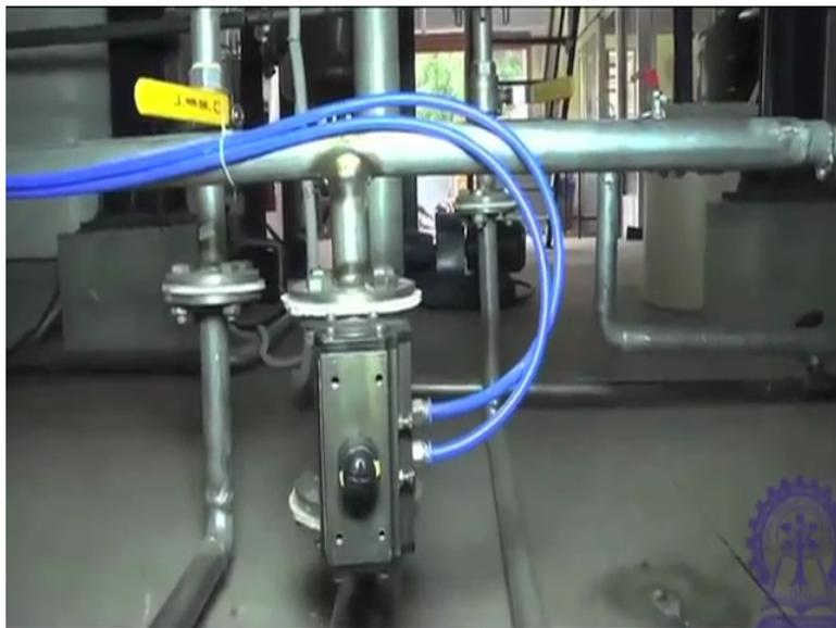
The feed in the feed preparation tank is transferred to various reactors with the help of pumps, in order to start the operation of the 10 metre cube reactor feed from the feed preparation tank is initially transferred to the feed tank 2 with the help of a centrifugal pump, nitrogen is passed in the feed tank 2 for sufficient time to maintain anaerobisity, this feed is further transferred from the feed tank2 to the 10 metre cube reactor.
